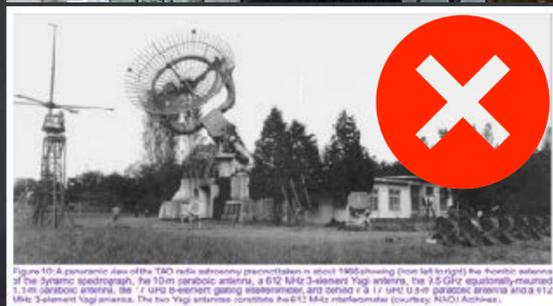
Figure 10: A panoramic view of the TAO radio astronomy precinct taken in about 1966 showing (from left to right) the Fourier antennas of the dynamic spectrograph, the 10-m parabolic antenna, a 612-MHz 3-element Yagi antenna, the 3.5-GHz equatorially-mounted 7.1-m parabolic antenna, the 11-UPS 6-element gating interferometer, and behind it a 1.1-UPS-U-ant parabolic antenna and a 612-MHz 3-element Yagi antenna. The two Yagi antennas constitute the 612-MHz interferometer (courtesy: NAOJ, Aoshima).
